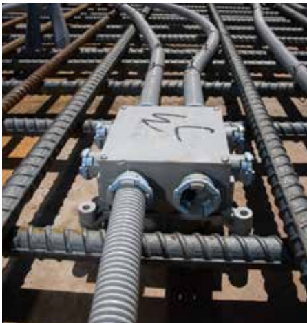
Westlake Slab Boxes Hubs are Elevated to Permit a Larger Diameter Rebar
