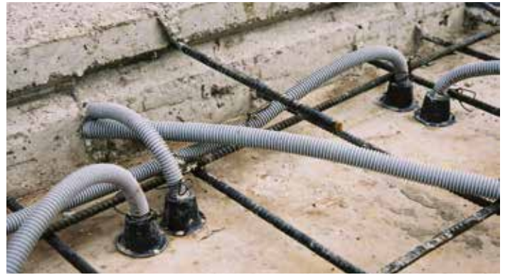
Diagram 2. ENT Encased in a Concrete Application
