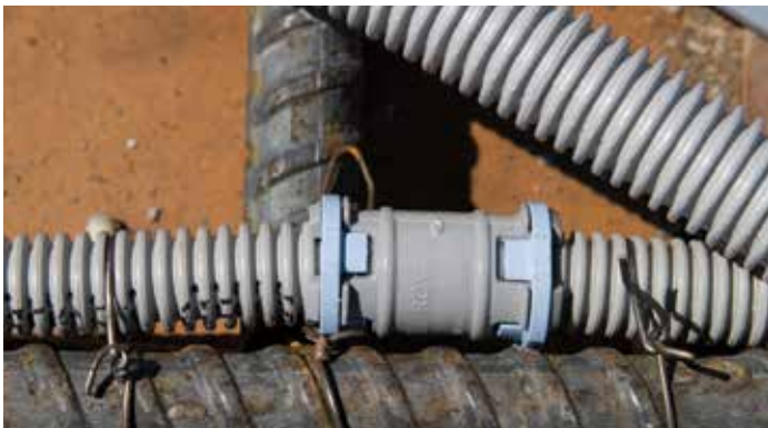
Diagram 1. ENT Pipe Attached with a Coupling and Tied to a Rebar
