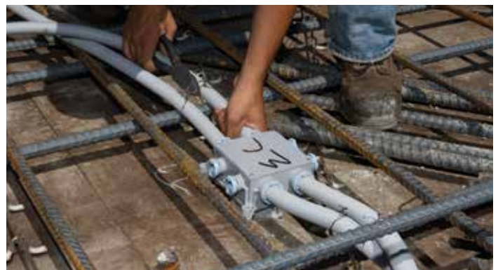
Diagram 3. ENT Pipe and Fittings in a High-Rise Application
