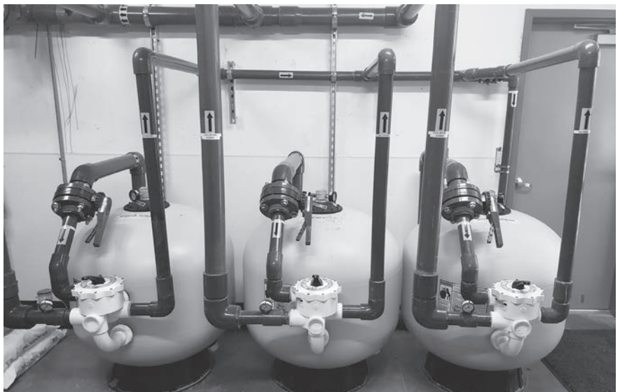
Commercial Pool system with Colonial BFVs
