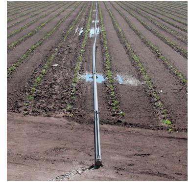
Aluminum System – Puddling Around Leaking Joints
