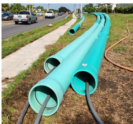
In the Gibsonton S2S Phase 1B project, the strategic use of HDD with segmental PVC along congested and high-traffic corridors minimized disruptions to the community while ensuring the safe and efficient installation of critical force mains.
