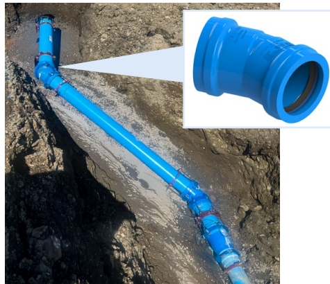
AquaConnect® AWWA C907 Molded PVC Fittings - 45° Elbow
