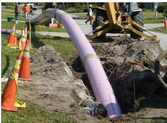
Installation of Certalok/RJ via HDD demonstrates the bending capability of a string of Certalok pipe segments while maintaining full integrity of the gasketed joint.
