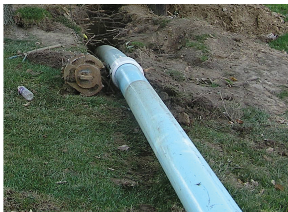
Installation of Certalok/RJ via HDD demonstrates the bending capability of a string of Certalok pipe segments while maintaining full integrity of the gasketed joint.
