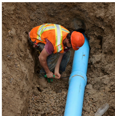
Spline insertion after installation
