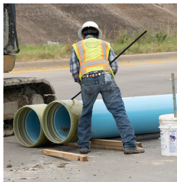
Spline insertion before installation
