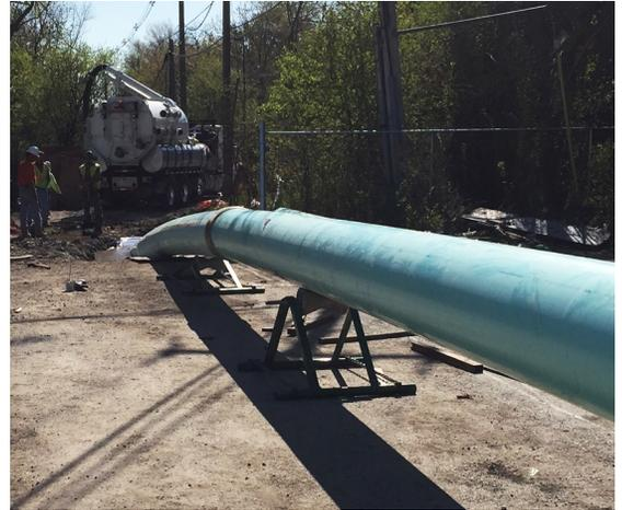
Morley said they chose Certa-Lok PVC pipe for its ability to hold up in the unstable ground of the wetlands. The easy-to-assemble restrained joints would also prove useful because the crew had limited space to assemble the pipe while working near the creek. The time-tested 18-inch Certa-Lok pipe was a perfect solution for this project.
