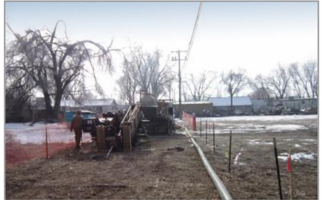
At the end of each ream, the crew attached the joints of 12-inch Certa-Flo pipe onto the drill head and the pipe string was pulled into place. The crew easily assembled the pipe, adding joint after joint as the pullback process continued. The crew used 10-foot joints in the more constricted sections and 20-foot joints elsewhere.
