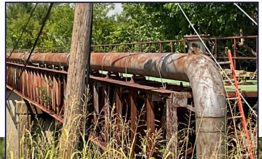
ORIGINAL STEEL WATER PIPELINE
