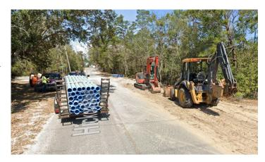
With the success of the project, Midway Water System has asked Evans Contracting to continue improving fire protection systems in other surrounding roadways with the installation of another 6000-8000 feet of Certa-Lok water main via HDD.
