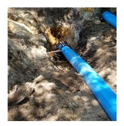
Typically, a fire protection line is designed with a larger diameter pipe, compared to the drinking water distribution pipes, to handle higher water flow rates. The pipes are connected or 'looped' through a series of valves and control points allowing the fire department to isolate the fire protection line. The looped configuration of the pipe ensures a constant water pressure and flow even in the event of high water demand.
