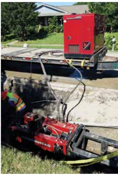
*Pipe bursting equipment has compact footprint. Installation was completed and service restored to residents on the same day*
